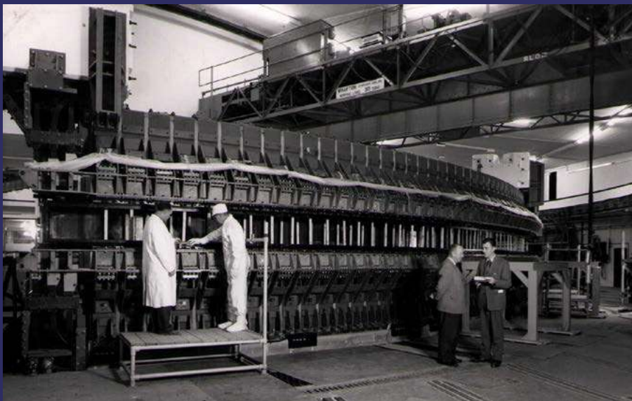
View of Nimrod octant with outer vacuum vessel installed. (1966)
