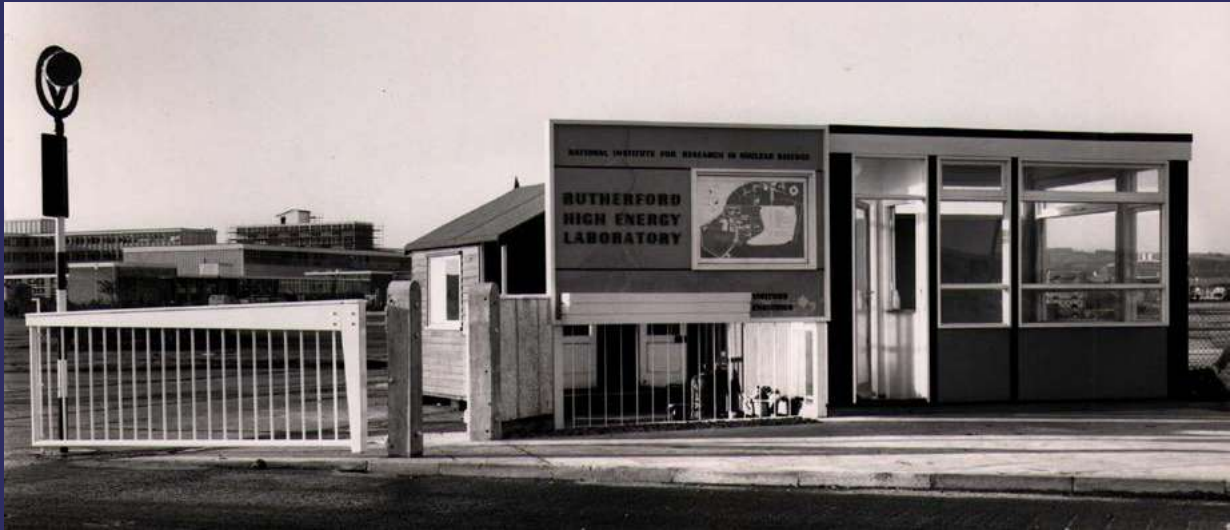
RHEL Main Gate. In the distance, Building R1 has been completed but R2 is still under construction and surrounded by scaffolding. (November 1963)
