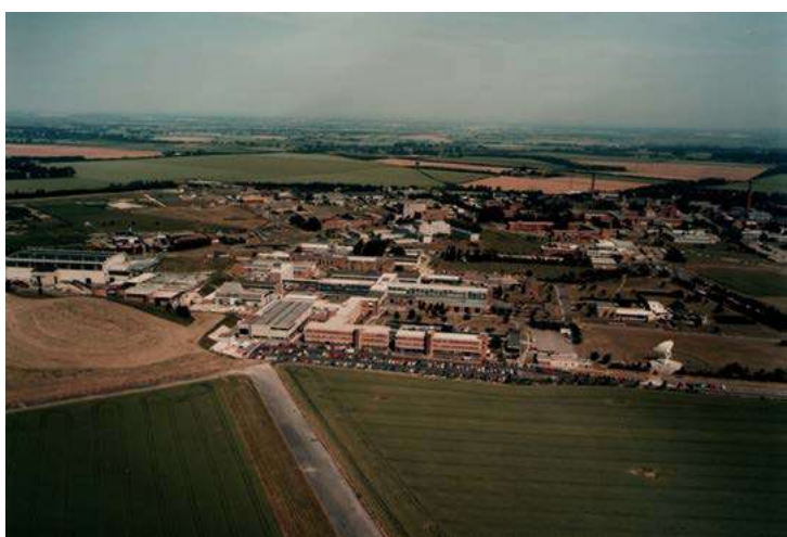
Aerial view of Rutherford Laboratory looking north. The NASA/IRAS satellite dish is in the right foreground with the R22 Restaurant further to the north. The hill covered in dried grass is Nimrod/ISIS spoil (this photo was taken in July); the accelerator mound itself is the green(ish) circle northwards. (1984)
