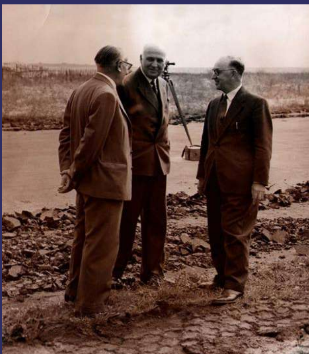
John Cockcroft inspects the Nimrod excavation work. (1957)
