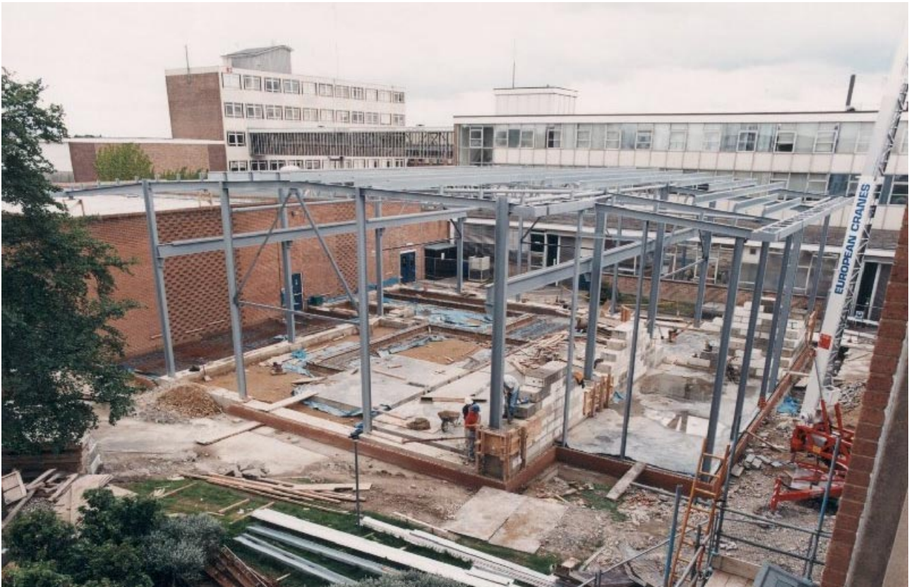
Photo 1. Building as at May 2000 - Foundations complete, steel framework erected, reinforced concrete plinths cast.
