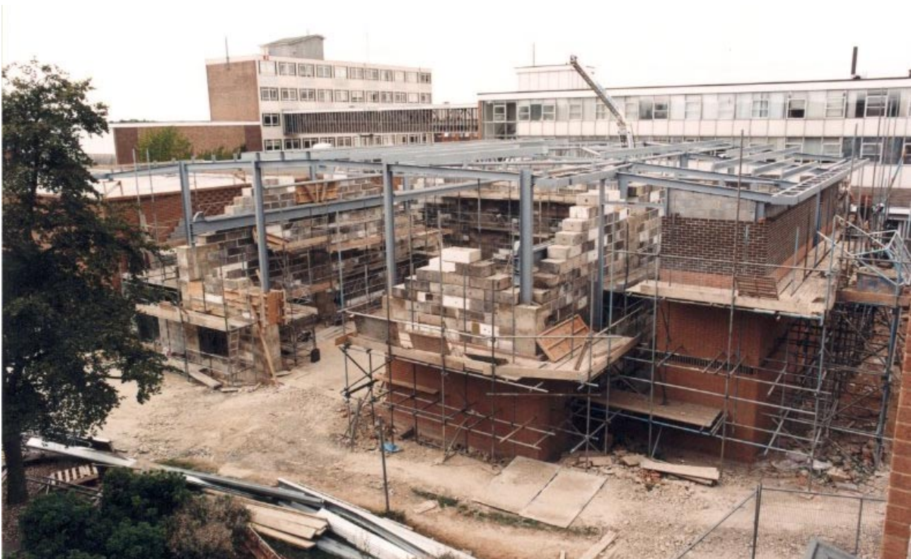
Photo 2. Building as at June 2000 – Floor complete, internal concrete shielding and external brick wall being erected.
