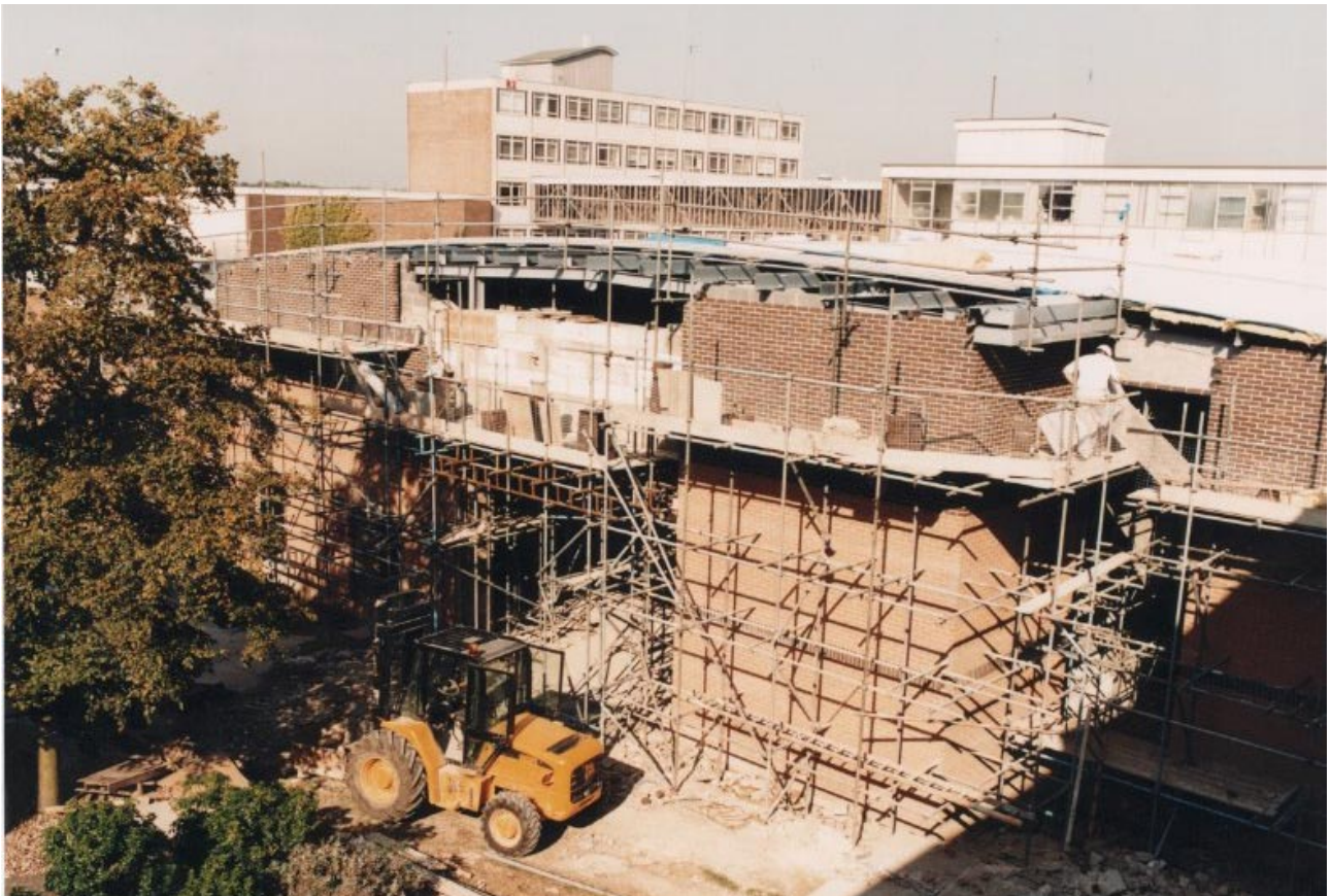
Photo 3. Building as at September 2000 – Internal concrete shielding and external brick wall nearly complete, crane installed, aluminium roof installed, building services plant being installed internally.
