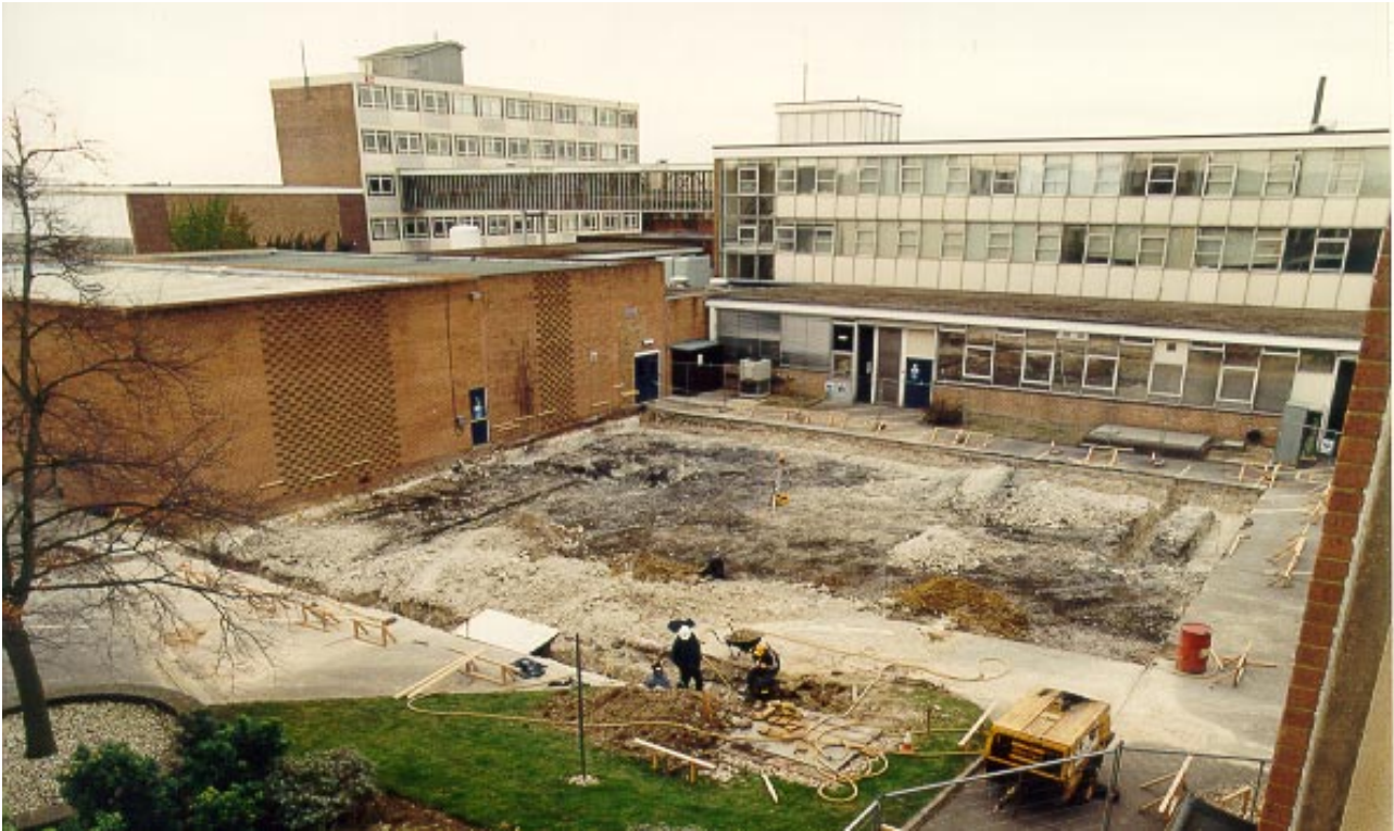
Figure 2. Progress on Vulcan Petawatt Building as at the end of March 2000.
